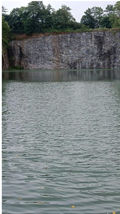
Rain Water Harvesting Pond
